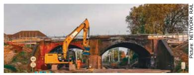
DEMOLITION DAY: The bridge over the four-track main line at Bedford was demolished in November to make way for electrification work north of Bedford on the Midland main line
