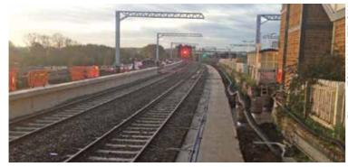
CONSTRUCTION: The footings for the down slow platform extension at Wellingborough station plus electrification work
